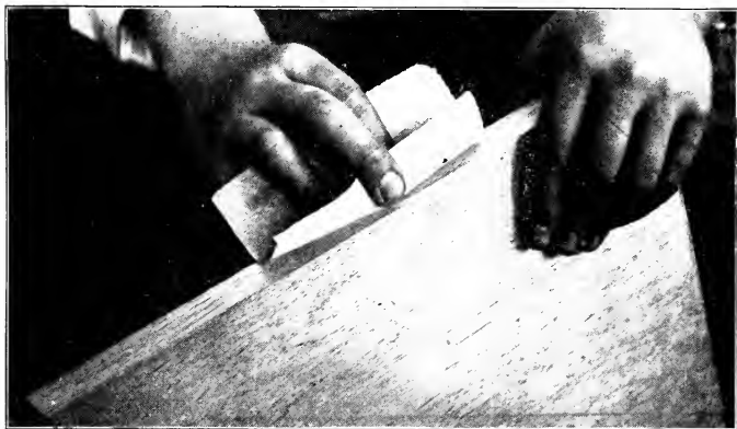
Fig. 123—Sandpapering Edge with Hand
